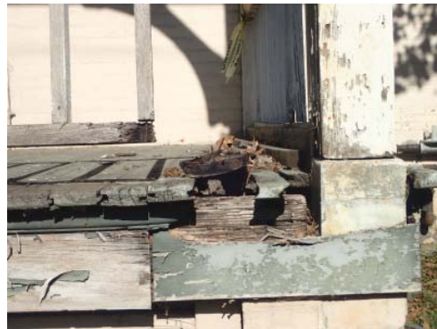
Photo PL10 Deteriorated wood framing at floor of South Porch
