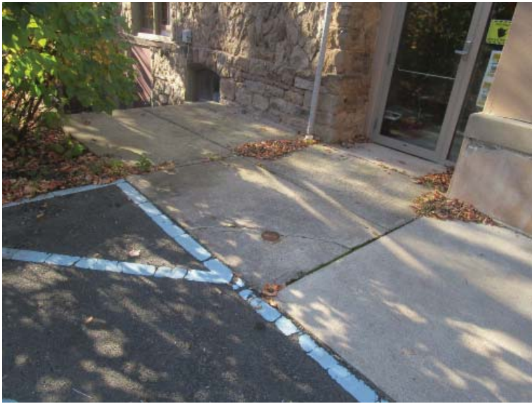
CRACKED SIDEWALK NEAR ADA ENTRANCE
