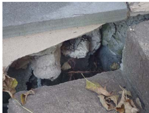
Photo PL 18 Closeup of settlement at stair
