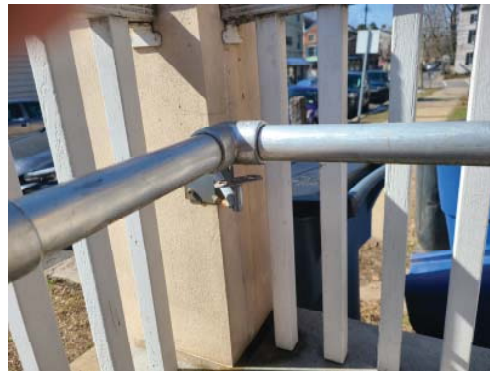
Photo PL 16 Loose handrail at handicapped ramp
