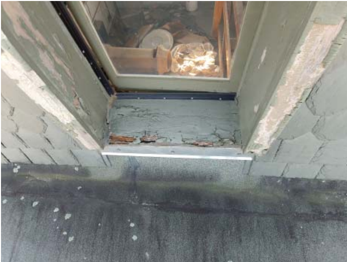
Photo 40 Photo is towards the cupola from the outside roof. The sill and trim needs to be repaired and repainted. The door needs to be watertight. The path to the door at the cupola interior needs to be cleared. The roof appears to slope towards the cupola instead to the perimeter drains that will continue to cause the potential of water infiltration around the cupola. The roof should slope away from the cupola.
