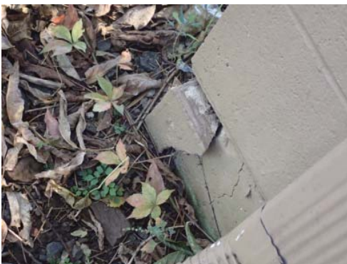
Photo PS 5 Damaged concrete masonry at southwest corner
