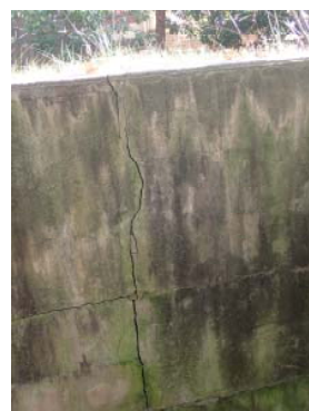
Photo CH8 Cracking in masonry wall at areaway
