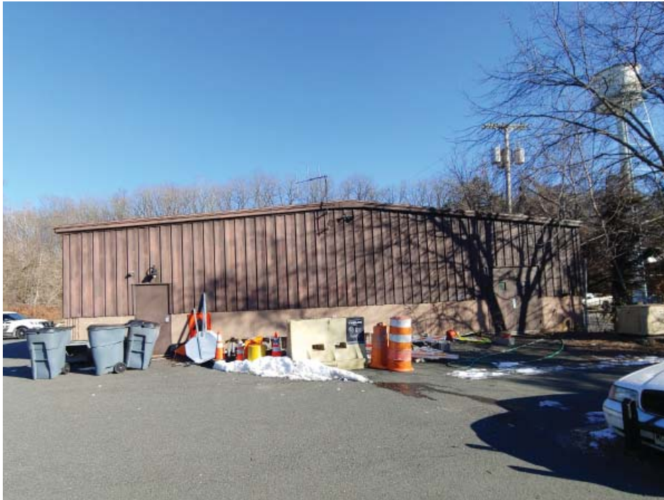
Photo 4 West façade. Repaint the metal siding and doors all around the building. Replace exterior lighting with LED lighting fixtures.
