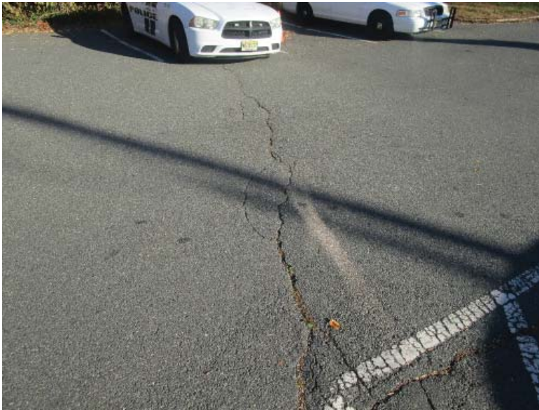
SPIDER CRACKS IN PAVEMENT
