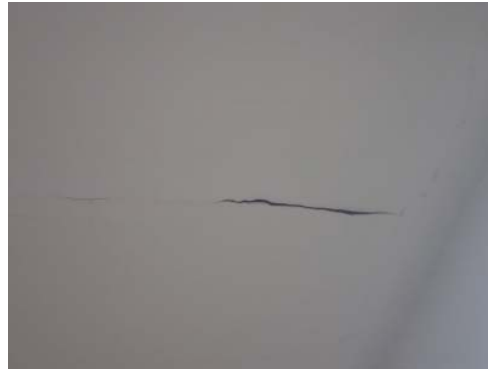
Photo CH10 Cracking in plaster second floor ceiling
