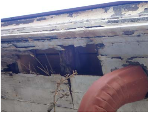
Photo PL 13 Deteriorated soffit at eave
