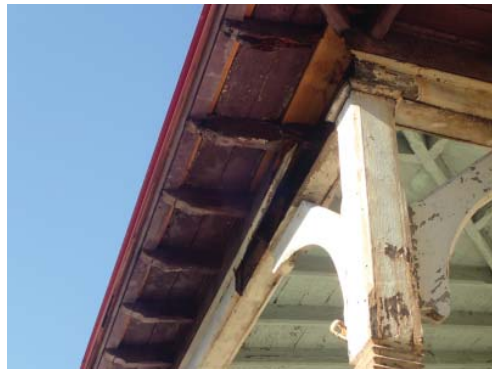
Photo PL 9 Deteriorated wood framing at eave of South Porch
