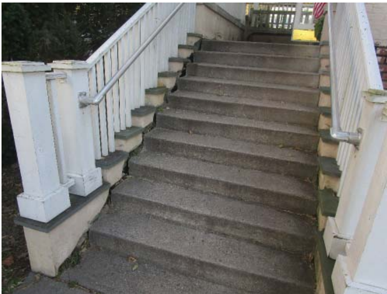
STAIRS SEPARATING FROM WALL
