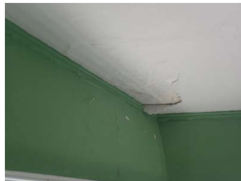
Photo PL24 Ceiling showing leaks.
