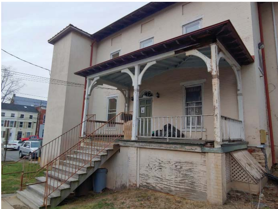
Photo 4 Back (South) facade. All surfaces need to be repainted. The plywood hatch cover at the right side of the porch needs to be replaced. Some of the porch floor planks and guardrail need to be replaced. Repaint the stair handrails. Repoint stone foundation wall, parge and repaint. Repoint masonry wall and repaint.
