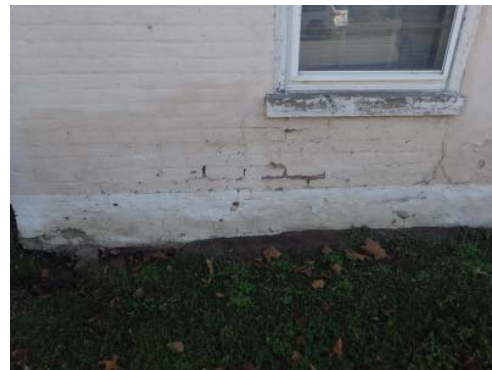
Photo PL 4 Washed out mortar in brick masonry
