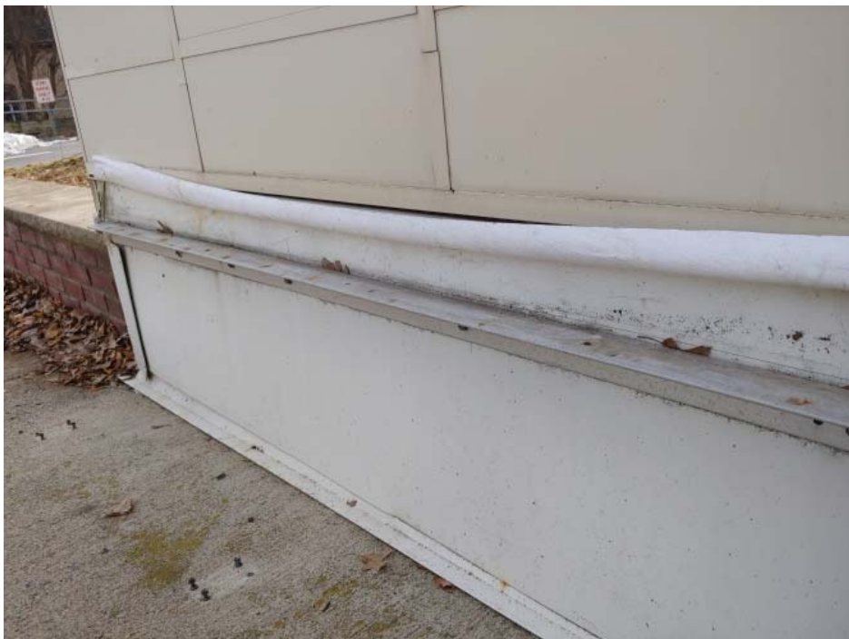
Photo 4 Trim missing over waterproofing at front (east) facade
