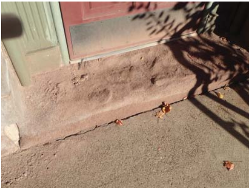
Photo CH5 Front stoop deterioration
