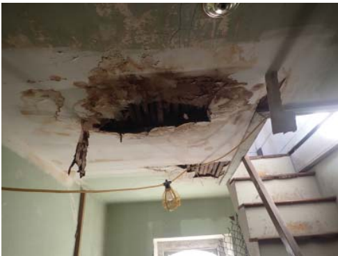
Photo CH11 Water damage failure of ceiling lath and plaster
