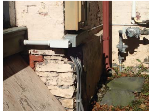
Photo PL-2 Deteriorated stone masonry mortar and parge coat
