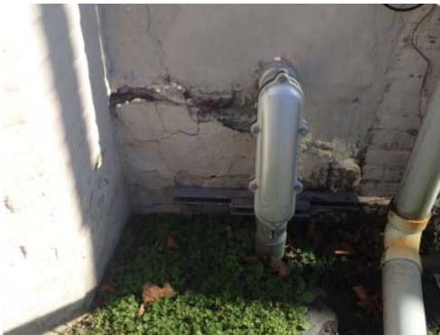
Photo PL21 Electric Utilities below flood elevation
