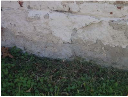
Photo PL 1 Deteriorated parge coat reception area (North)
