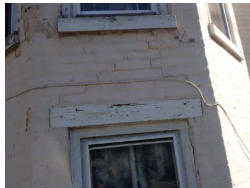
Photo PL6 Break Room Window 2 nd Floor note settlement cracks
