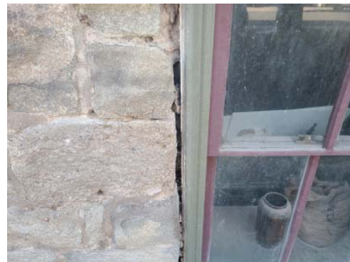
Photo CH2 Separation of window frames from masonry
