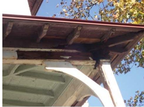
Photo PL8 deteriorated wood framing at eave of South Porch
