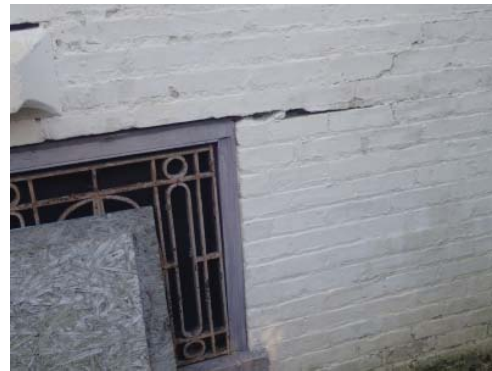
Photo PL 22 Wall opening below flood elevation
