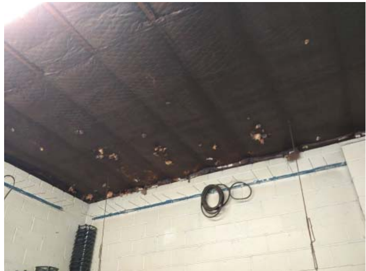
Photo 15 Replace damaged insulation in the ceiling of the Garage Room 001.
