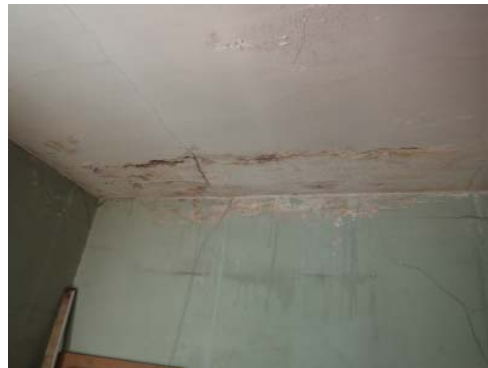
Photo CH12 Water damage failure of ceiling lath and plaster
