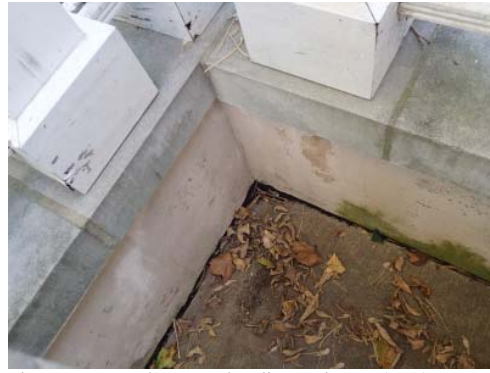
Photo PL 14 Settlement at handicapped ramp (East)
