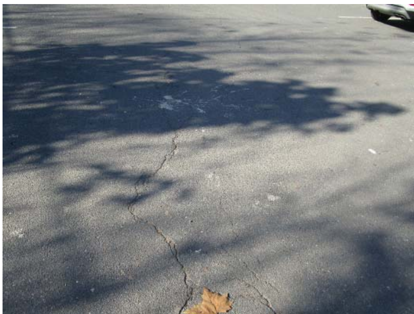
SPIDER CRACKS IN PARKING LOT
