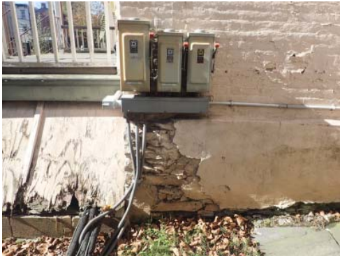
Photo PL19 Electric Utilities below flood elevation
