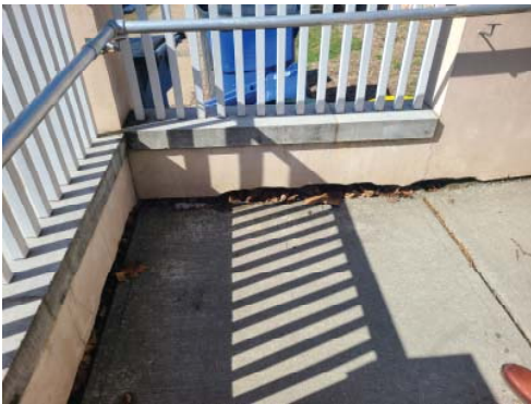
Photo PL 15 Settlement at handicapped ramp (East)
