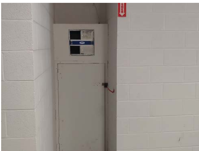
Photo 49 Replace missing fire extinguisher in the Sally Port 005.
