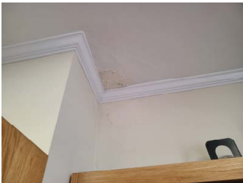
Photo PL 25 Water leak at ceiling
