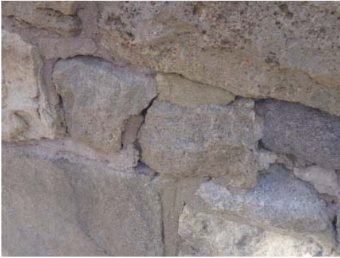
Photo CH3 Deterioration in exterior stone masonry cladding
