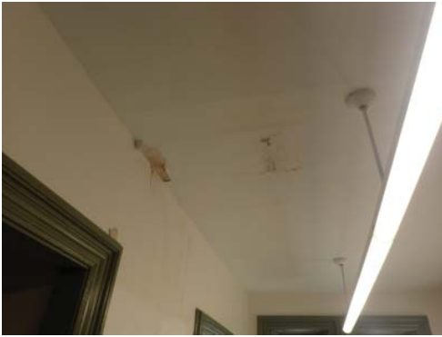
Photo CH9 Cracking in plaster second floor ceiling
