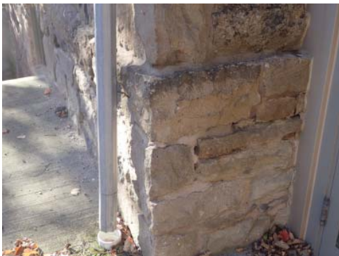
Photo CH1 Cracking in exterior wall
