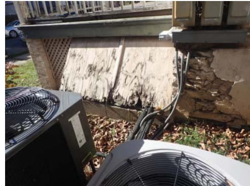
Photo PL 20 HVAC and wall opening below flood elevation
