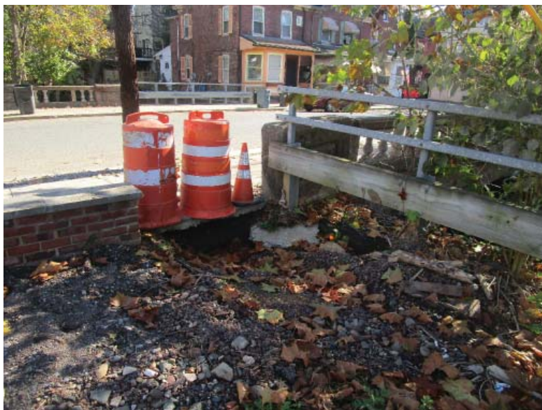
WASHOUT NEAR PARAPET WALL
