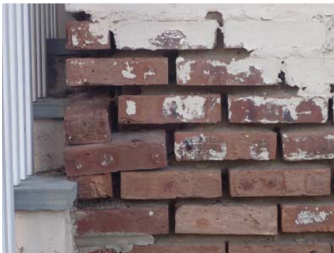
Photo PL 3 Washed out mortar in brick masonry
