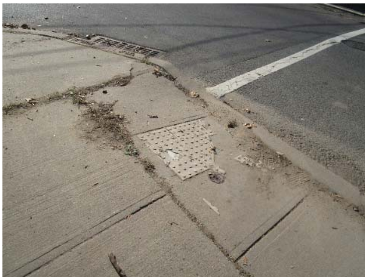
DAMAGED DETECTABLE PADS
